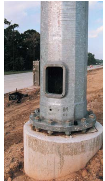
Shown here is the area the RKI winch is installed in the light pole.
